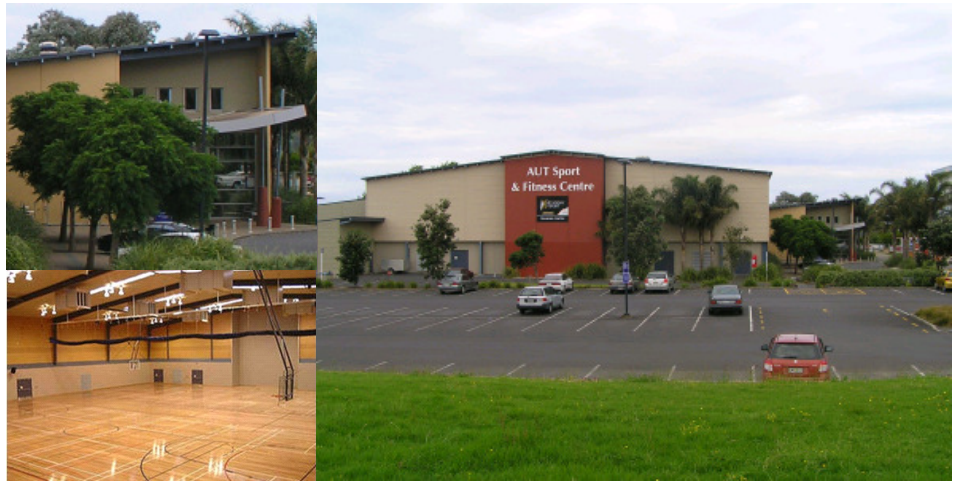
Entrance foyer (top left), sprung wooden floor (bottom left), exterior and car park (right)
